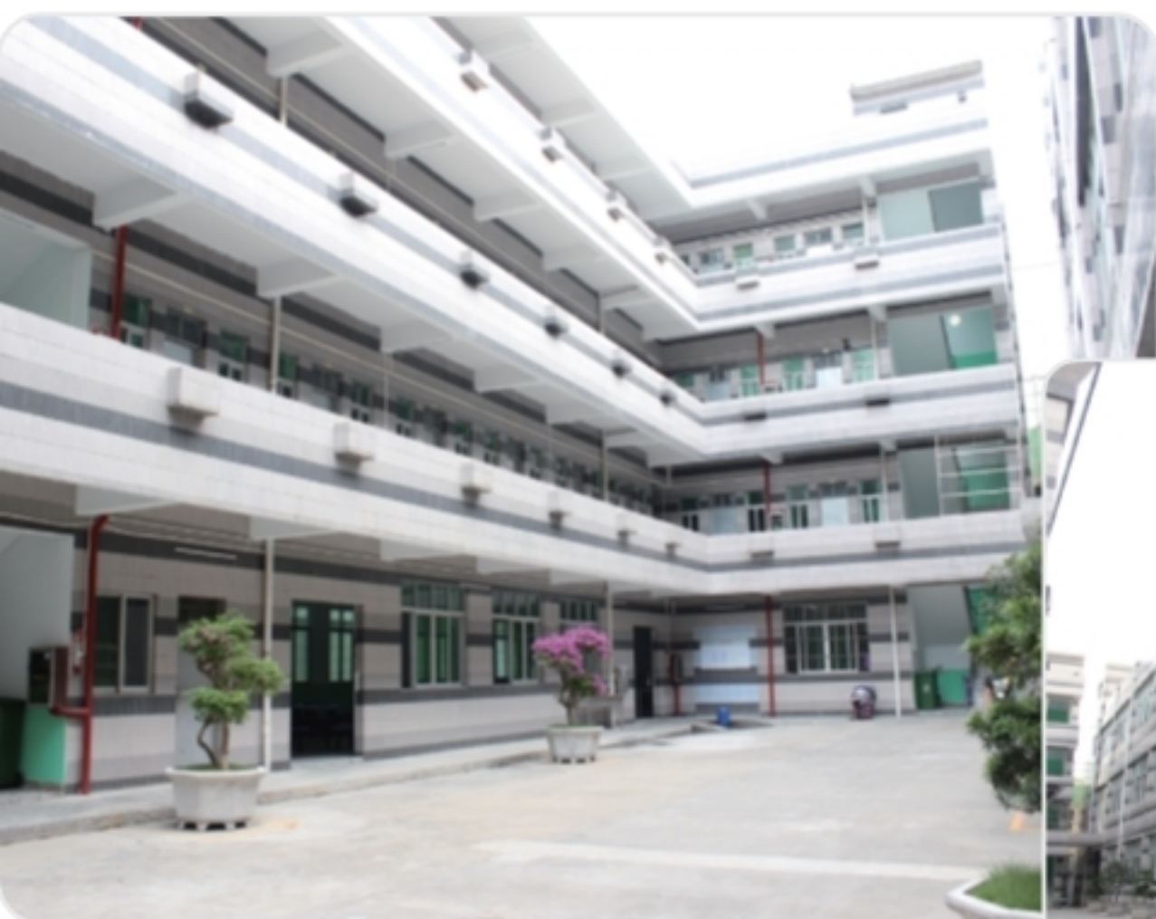
廠區1/The factory
